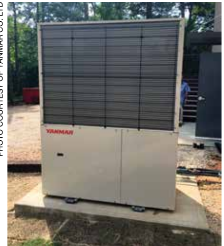
STAE implemented Yanmar's Variable Refrigerant Flow (VRF) technology at its new office near Auburn City in Lee County, Alabama.
