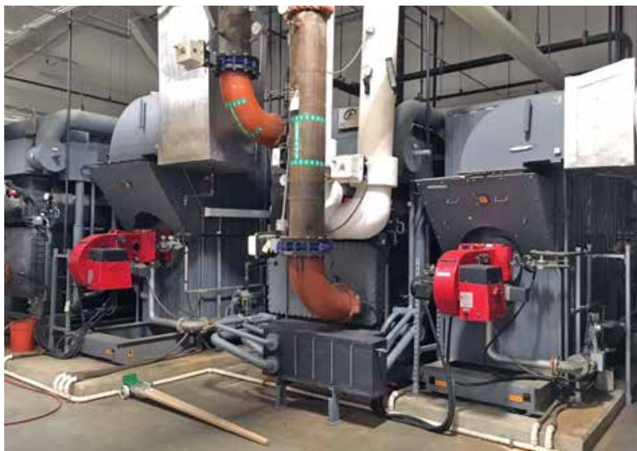
The Jordan Furniture facility is cooled and heated by 739-ton and 537-ton, direct-fired absorption chillers by Broad U.S.A. that burn natural gas and convert it to chilled water for air conditioning.
