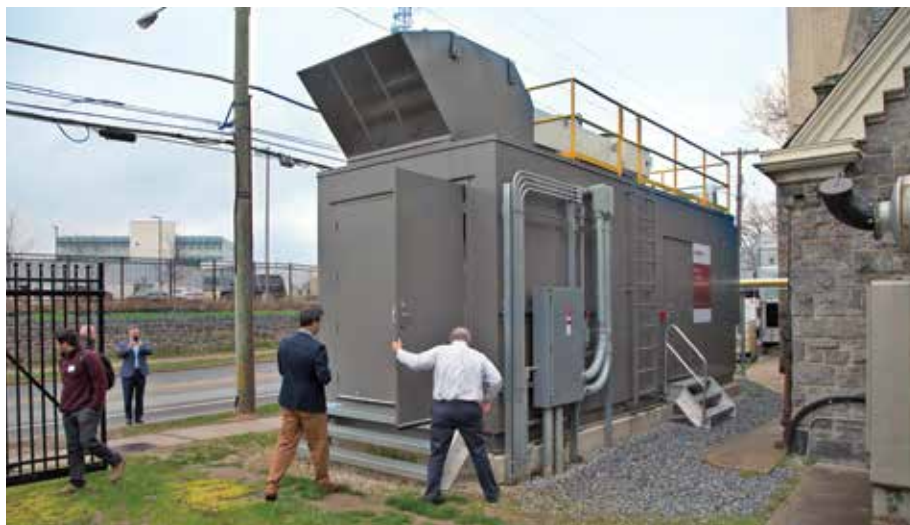
Cathedral Village replaced failing equipment with a high efficiency 265 kW natural gas engine by ENER-G Rudox to provide heat and electricity.
