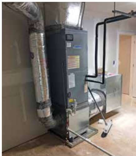
The STAE group of contractors deployed one, 12-ton natural gas-powered, VRF system which was connected to three 4-ton air handlers for both heating and cooling.
