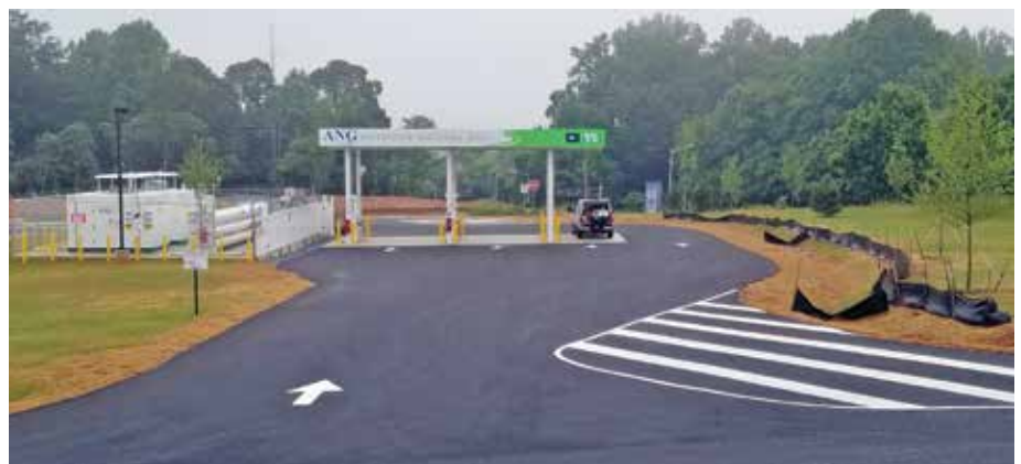
Frito Lay just added a fast-fill compressed natural gas fueling station in Lynchburg, Virginia, operated by American Natural Gas LLC.
