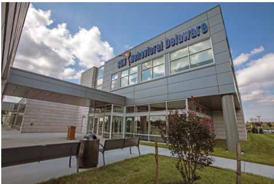
SUN Behavioral Delaware’s new 90,000-square-foot facility uses natural gas to fuel heating, water heating and cooking.
