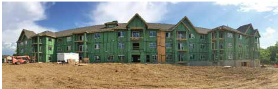
The Village Cooperative in Kansas City, Missouri, (seen here under construction) is another multifamily project preferring natural gas to electricity for heating. Each unit at the Village Cooperative has a natural gas Magic-Pak by Lennox for space heating.
