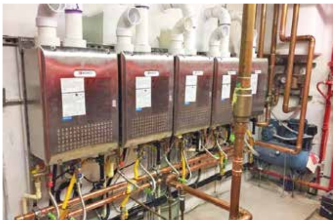
A bank of five Noritz condensing tankless water heaters are installed in a mechanical room at one end of each of the five buildings making up the 250-unit multifamily Spanos Corp. complex in Sanford, Florida. The design saves $800 per unit, or $200,000 in upfront costs.
