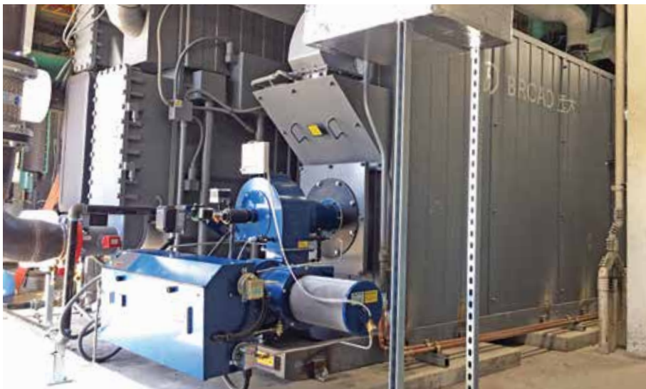
The Rock Church campus boiler room was fitted with direct-fired absorption chiller from Broad USA Inc. to burn natural gas and convert it to chilled water for air conditioning.
