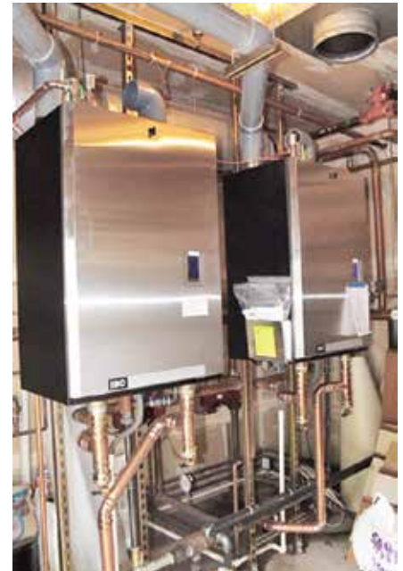
PHOTO COURTESY OF LOCKHEED MARTIN/CASCADE NATURAL GAS CORP.
