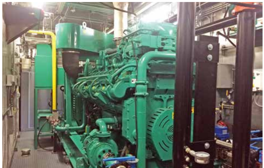
A 1.1MW Cummins natural gas-fired reciprocating CHP system provides about 75 percent of the daily energy needs for Eastern Regional Medical Center, one of five hospitals in the Cancer Treatment Centers of America network. The CHP system also provides up to 90 percent of the center's heating needs.
