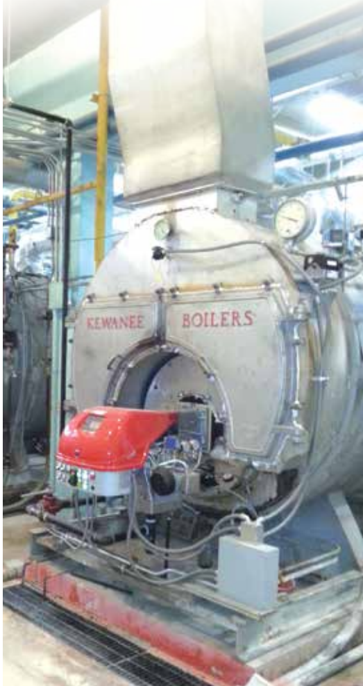
Older serviceable boilers can be equipped with advanced burners to improve boiler turndown, reduce excess air and reduce emissions. Often efficiency gains of 5% to 30% are achievable. Photo courtesy Riello Burners.
