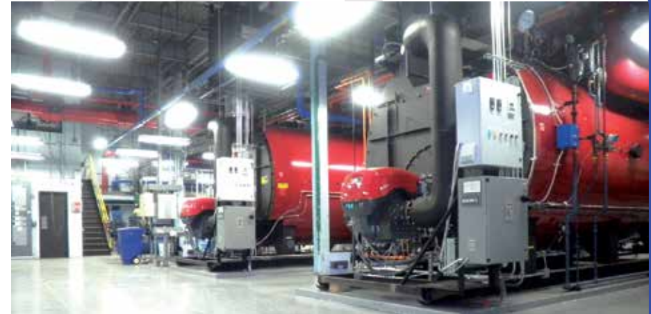
Facilities with multiple boilers especially benefit from burner replacement where they can be linked to central plant control to allow boiler optimization for varying plant loads. Photo courtesy Riello Burners.
