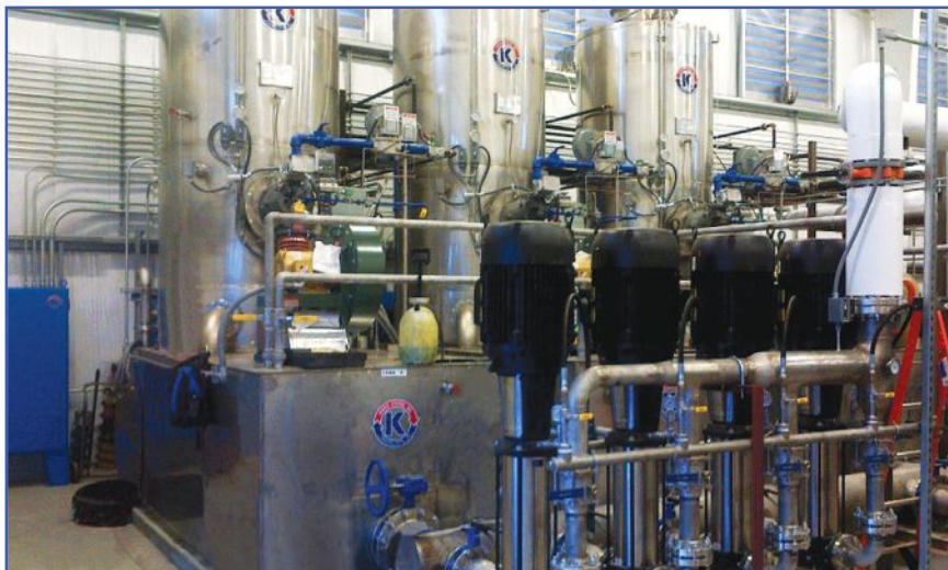
For installations requiring very large volumes of hot water, multiple units can be installed. Photo courtesy Kemco Systems.
