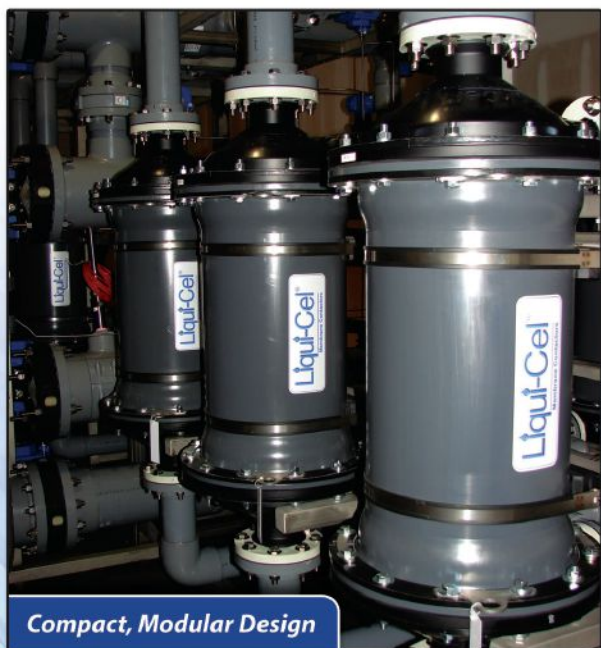
Compact, Modular Design 14-inch Industrial Deaeration System
