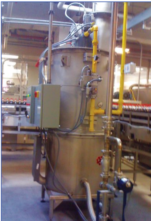
This direct-contact water heating unit is installed on the floor of a bottling plant, the type of industry that needs plenty of hot water for washdown and sanitation. Photo courtesy Armstrong International.
