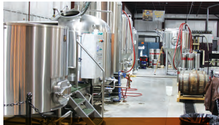
Microbreweries can reduce energy use by heat recovery from the brewing process, selecting high efficiency electrical machinery, and by use of an efficient gas-fired low pressure boiler. Photo courtesy: Rick Staszewski.
