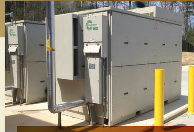
The Sierra Nevada brewery in North Carolina uses biogas from wastewater treatment to fire these microturbines for plant power supply. Photo courtesy: Sierra Nevada Brewing Company.
