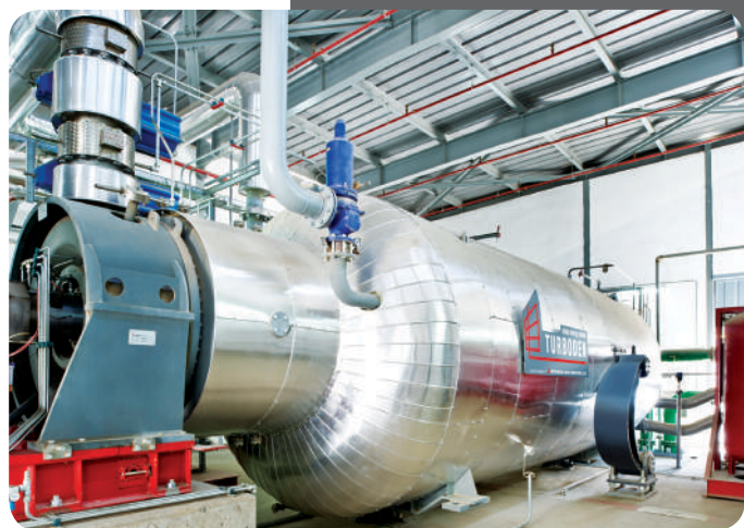
A view of an installed Turboden ORC heat recovery application for electric generation. Photo courtesy: Turboden
