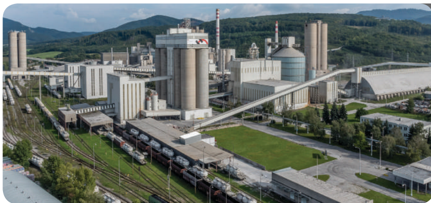
An organic Rankine cycle plant is used for heat recovery and electric generation at this cement manufacturing plant in Morocco. Photo courtesy: Turboden
