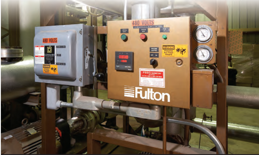
Controls on thermal fluid heaters integrate easily with central process controls.
