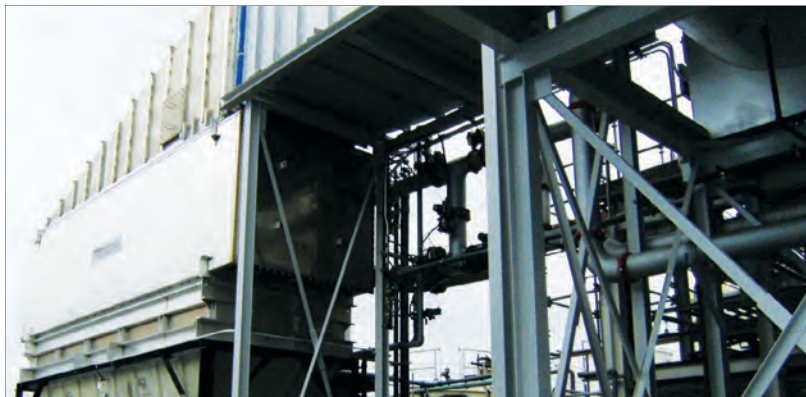
Economizers are a time-honored method of extracting useful waste heat from exhausts of boilers, gas turbines and industrial furnaces. Newer designs include condensing economizers and hybrid designs with both condensing and non-condensing sections. Courtesy: Condex.
