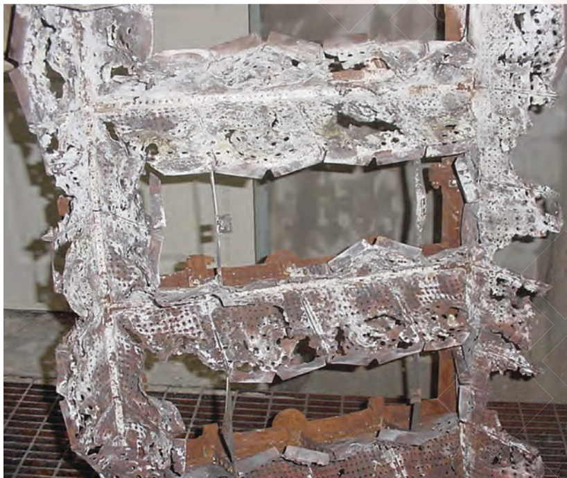
Regular inspection by trained employees or contractors will spot a wide range of burner problems, such as this severely corroded burner. Often the problems may be more subtle, such as wiring or control deficiencies or outdated control software. Courtesy: CEC Combustion Safety.
