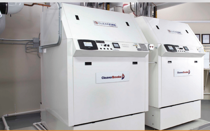
With cool return water temperatures, condensing hydronic boilers such as these Cleaver Brooks units offer efficiencies of 90% and higher. Photo courtesy: Cleaver Brooks
