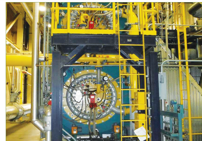
New burners extend the life of a dual fuel (natural gas & oil) boiler at the University of Wisconsin. Photo courtesy: Cleaver Brooks
