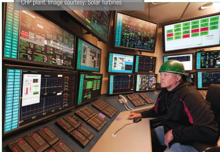
The central control room for Cornell University’s CHP plant. Image courtesy: Solar Turbines
