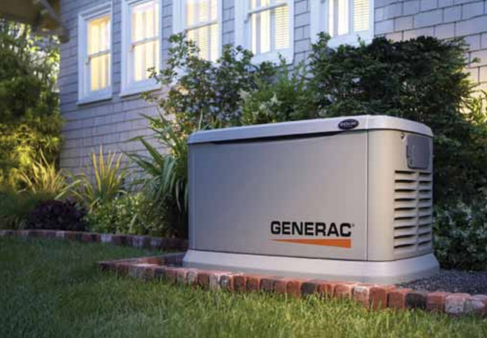
PHOTO COURTESY OF GENERAC
