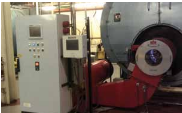
Northwest Community Hospital in Chicago replaced its burners before the end of their life cycle as a money-saving measure.
