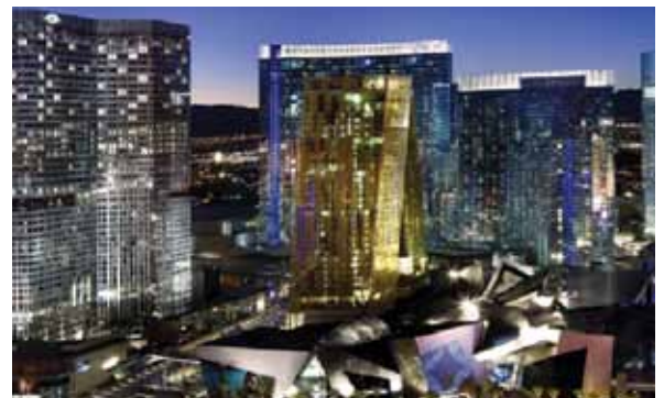
CityCenter in Las Vegas features an efficient, state-of-the-art combined heat and power (CHP) system.
