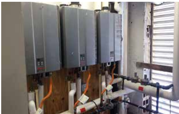
The Rinnai Tankless Rack System, featuring three natural gas tankless water heaters, was installed in the 16-story Thomas Jefferson Tower. The installation drastically reduced electrical system needs by 5,000 amps as well as decreased cost, space and maintenance requirements in the historic building.
