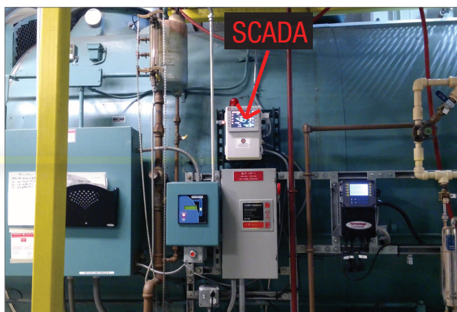
Lumec AOCS installed on a 700 bhp boiler at a medical facility in Kansas City. This project demonstrates the minimal modification typically needed to improve the efficiency of the boiler.
