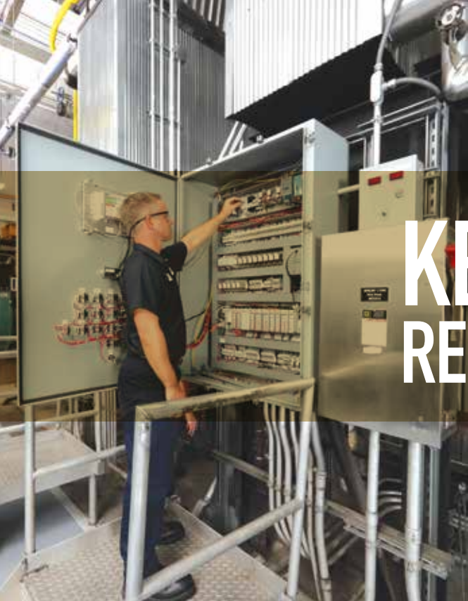
Today's boiler burner controls are sophisticated and allow a wide range of options, including using boiler exhaust gas analysis to optimize combustion. Photo courtesy Cleaver-Brooks.
