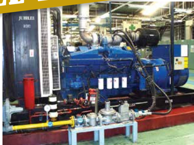
This Cummins engine has been retrofitted with a GTI-Altronic conversion system to allow simultaneous operation on diesel fuel and natural gas, thereby lowering the operating cost and reducing the on-site fuel storage requirement. Photo courtesy Altronic LLC.
