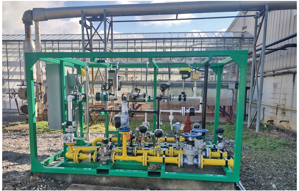
.PHOTO COURTESY OF NATIONAL FUEL GAS DISTRIBUTION CORP.
