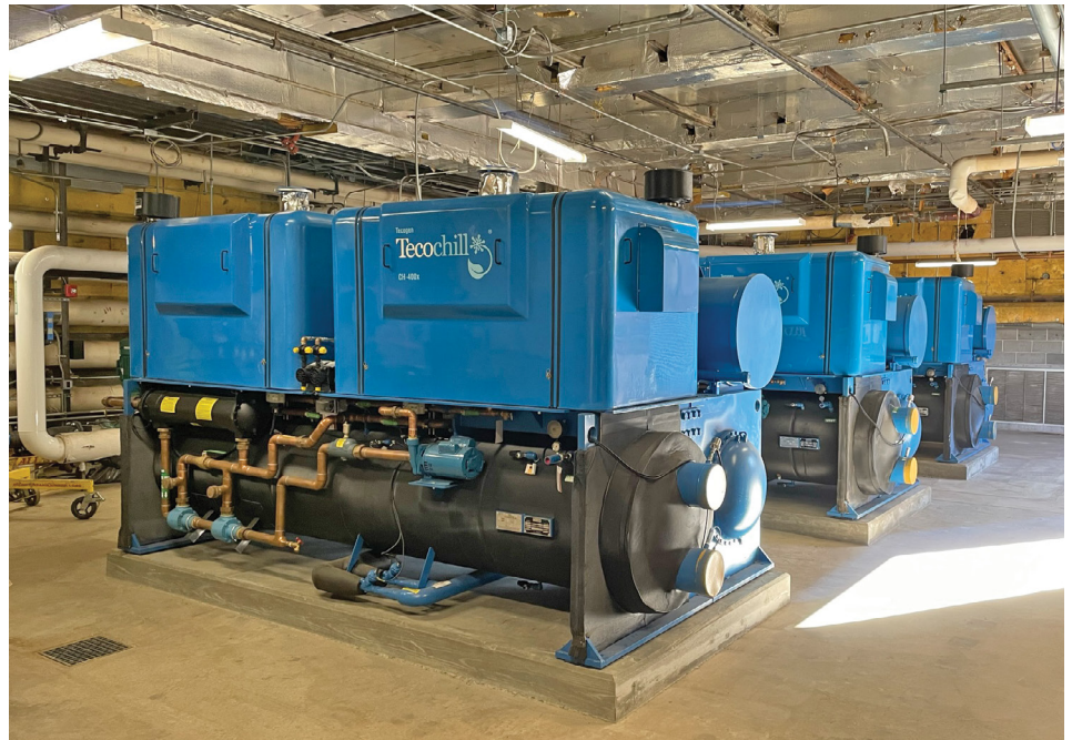
■ Greenwich High School in Greenwich, Connecticut, uses Tecogen Inc. natural gas engine-driven chillers to provide 1,400 tons of cooling at the school.
